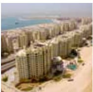
UAE, Dubai, Palm Jumeirah Luxury residential building in Palm Jumeirah Comelbus System 1.323 color Videocom monitors complete with CCTV system
